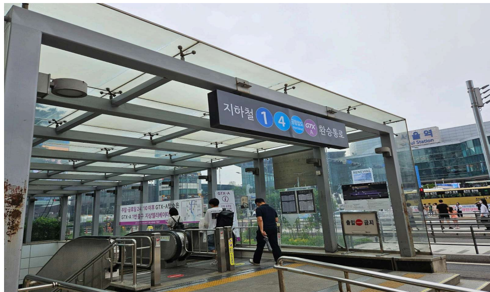
Figure 12. Entrance to GTX-A, Lines 1 and 4 at Seoul Station.
