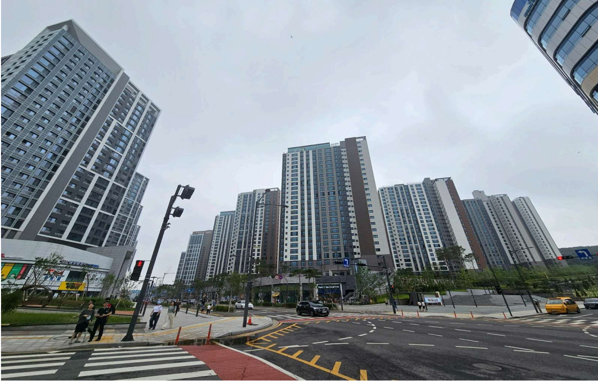
Figure 25. Geomdan New City in front of Singeomdanjungang Station.
